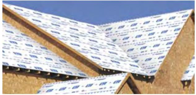
**ShingleLayment** is a lightweight, woven polypropylene underlayment coated with a non-skid TPO (Thermoplastic Olefin or Polyolefin). It has a very high tensile strength that resists tearing, ripping and blow-off from high wind exposure.
