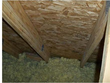
These insulation baffles (pictured above are ineffective since they are misplaced and damaged from heavy condensation. The baffles should be rigid and placed as shown (picture below) to keep wind from blowing under the insulation.
