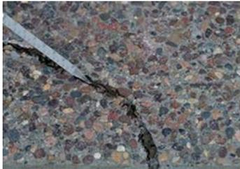
For typical slab-on-ground construction, there are two options for controlling restrained-shrinkage cracks. One consists of tooling or saw cutting contraction joints into the slab. Sometimes called control joints, these joints are actually weakened sections that crack and open to relieve the restrained-shrinkage stresses. The other consists of installing steel reinforcement to control the width, not the location, of the cracks. Combining both options can provide excellent crack control.
