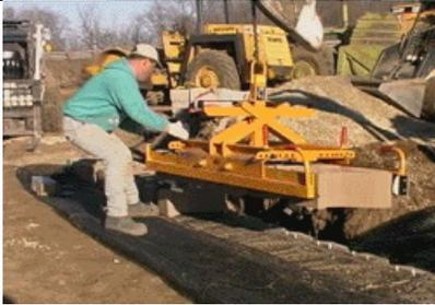
Retaining Wall Clamp speeds installation by up to 30 - 40 %
