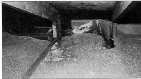
The insulation baffles pictured above are ineffective since they are misplaced and damaged from heavy condensation. The baffles should be rigid and placed as shown in the picture below to keep wind from blowing under the insulation and causing condensation, mold, and mildew at the ceiling corners.
