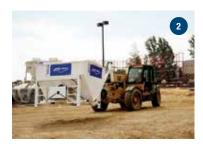
STEP 2: Move the SPEC MIX PA4000 Power Auger Delivery System to the desired location. Make sure the ground is level and stable. Place foot pads under silo feet. Silo height can be adjusted by lifting with a forklift and moving the pins that run through the silo legs.
