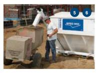
**STEP 5:** Place the mixer under the discharge auger and start mixer. Place water into the mixer.
