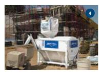
STEP 4: To load the PA4000, grab and pull back on handle for the top cover. Using a lift, hoist the bulk bag above either open cover. To open the bag, stand on ground while using a bag hook to open the bag chute. Once loaded, close covers. Stay off the top of the silo.
